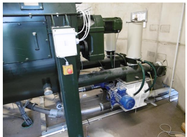
Pneumatic feeding system to the burners
