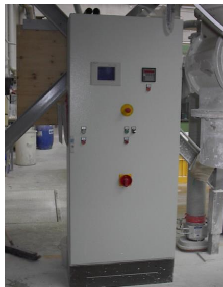
Control Board (totally new)
